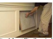
Step 3. Insert filter if required If your system requires a filter at the return air grille, insert your filter now. Remember - Top Goes in First (TGIF)!
